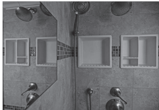
Figure 5. Grout around the mirror to seal and finish.
